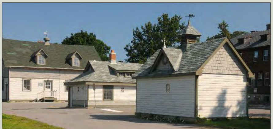
Behind the Genetics Building is a delightful set of service buildings that could quite conceivably still house clutches of pedigreed White Leghorn, Barred Rock or Rhode Island Reds, just out of their incubators.
